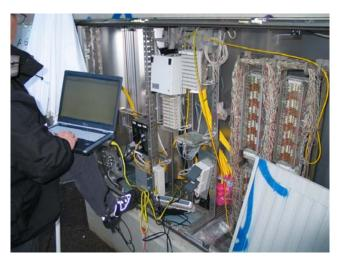
Service technician in the field: maintenance work on a switchgear panel
